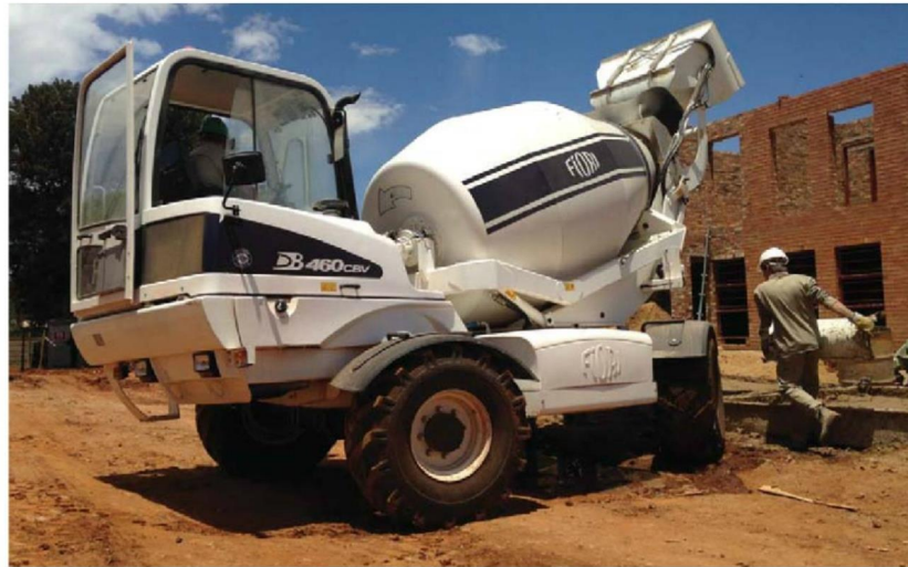
Fiori self-loading concrete mixer working on site.
