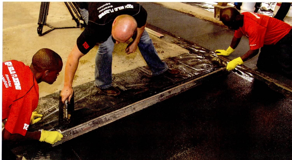
Stoneflow being placed by Rock Solid Flooring during a training session.
