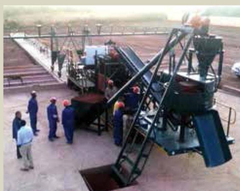
VB1X plant with bagbreaker and gantry on site in the DRC.
