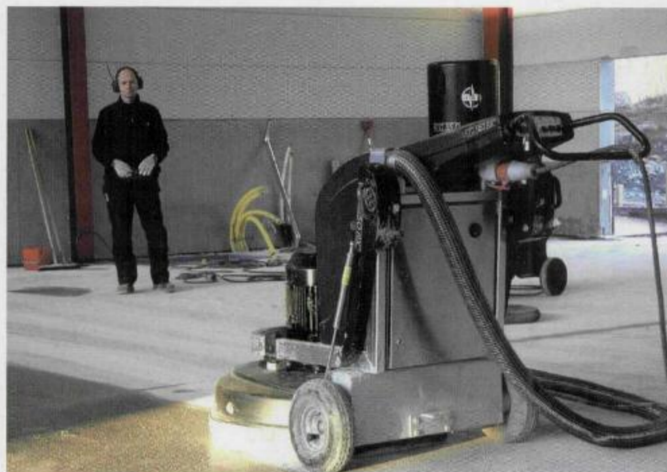
The radio-controlled HTC 950 RX is ideal for grinding large areas, and built-in dust extractors ensure that work can be carried out more safely and efficiently
