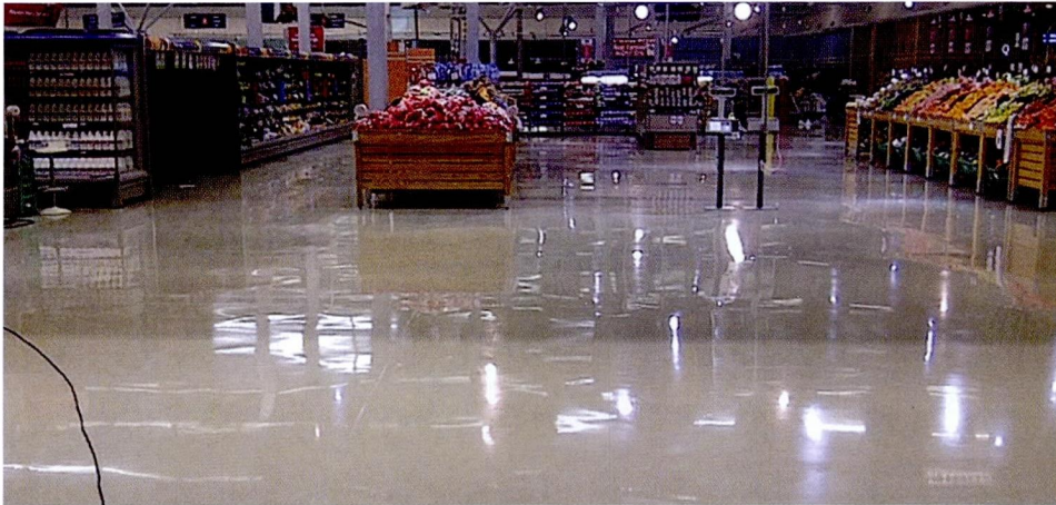
DCS Green Twister pads were used for burnishing the Hypermarket floors, resulting in a high gloss finish
