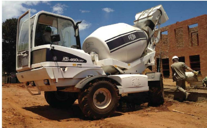
Fiori self-loading concrete mixer working on site.
