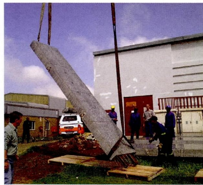
Use of an existing steel structure on the premises to create the PMSA showroom using pre-cast and pre-polished tilt-up concrete inner walls
